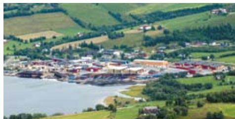
The Kjeldstad manufacturing facility, near Trondheim, Norway
