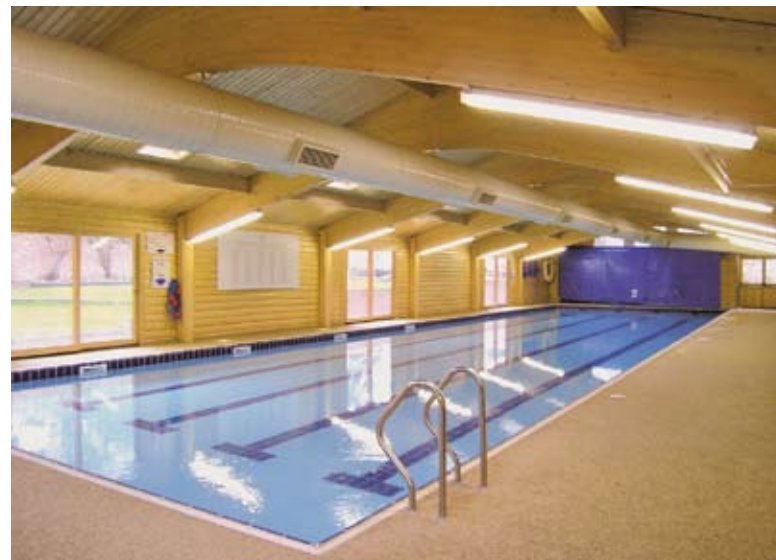
Indoor swimming pool, Cumnor House School, Haywards Heath, Sussex. Pool by Fowler Swimming Pools Ltd.
